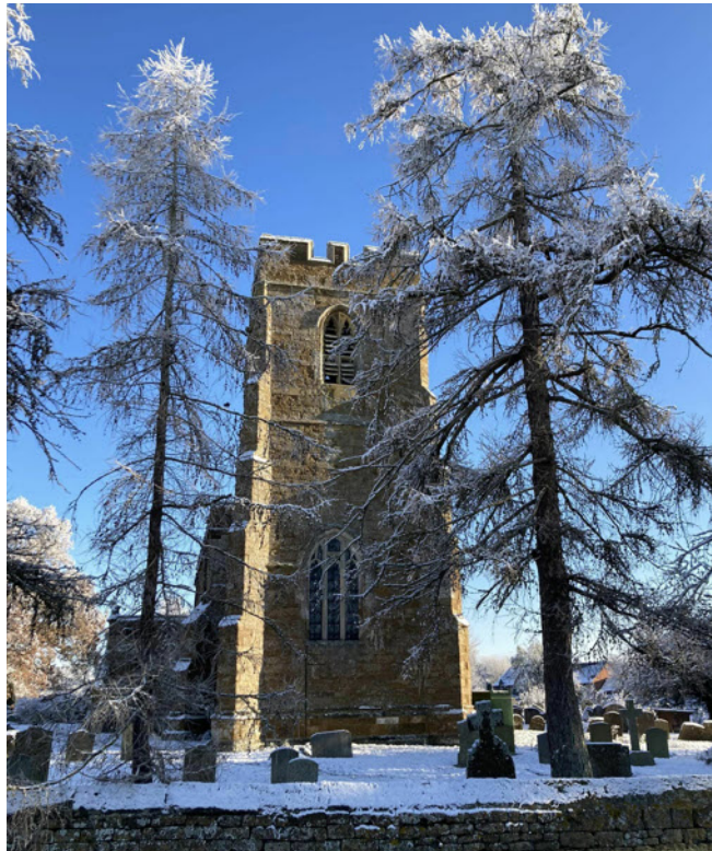
St Lawrence Church in December 2022. Photo by Tricia Harbour
